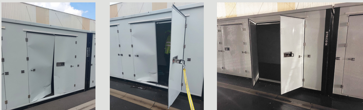
Replacing a severely damaged door due to a lorry accident
